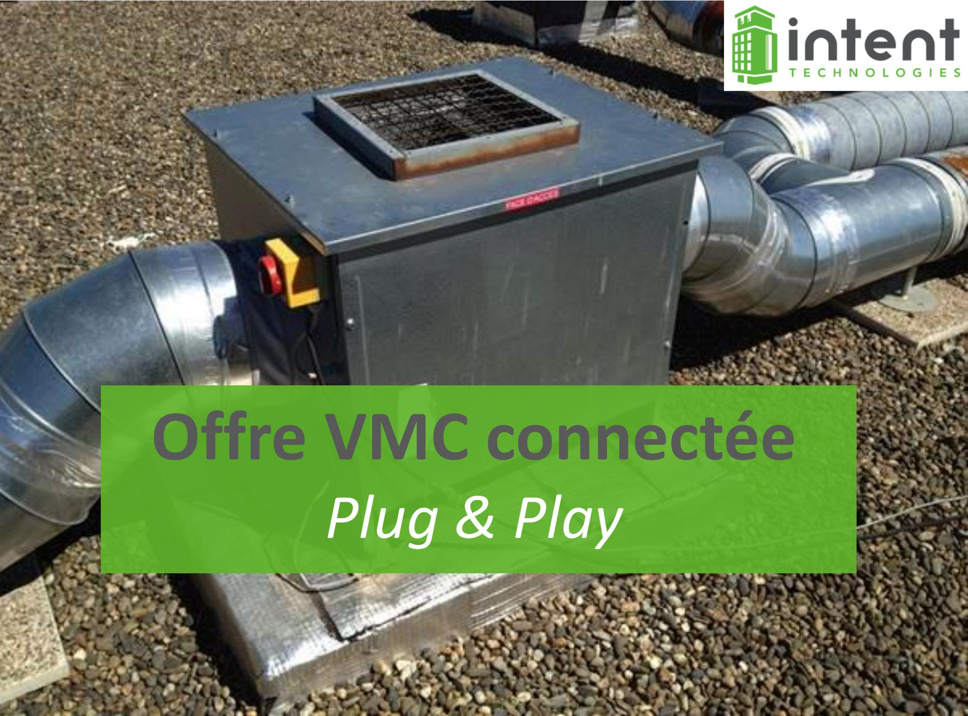
A photograph of a mechanical ventilation with heat recovery (VMC) unit installed on a roof. The unit is a dark grey metal box with a square air filter on top. It is connected to several large, insulated metal ducts. The roof surface is covered in gravel. A green banner is overlaid on the bottom half of the image.
